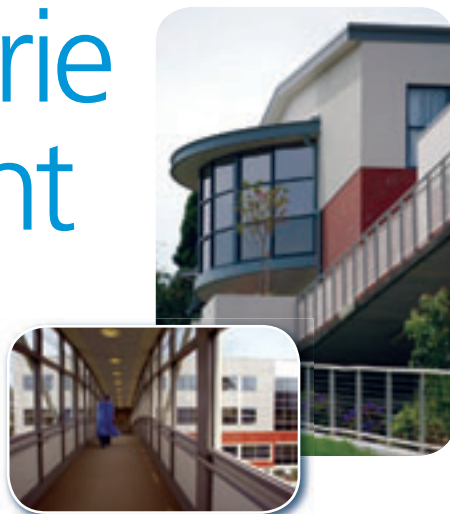
Above: The newly constructed Medical Centre & bridge link.
